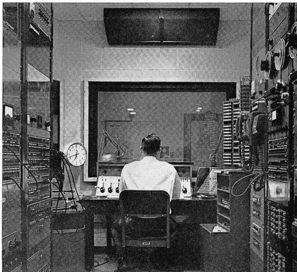
FIG. 29. Radio master control looking into Studio C.
