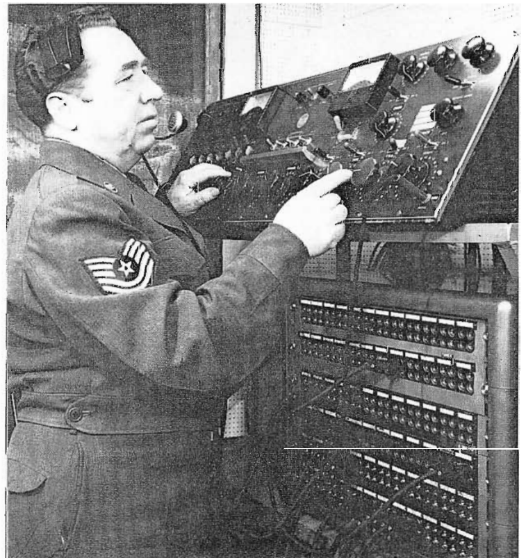
FIG. 12. Control room equipment includes dual channel audio console Type BC-7, permitting simultaneous use of two sound channels.
